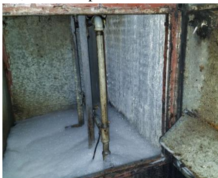
Figure 3: HRU washdown section showing clean coil.
